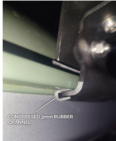
Figure 7: Completing gutter mount fitment
